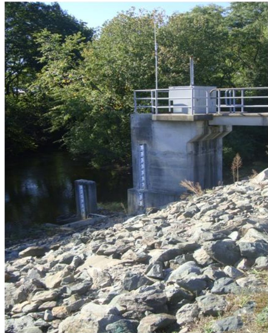
River Level Monitoring Station
